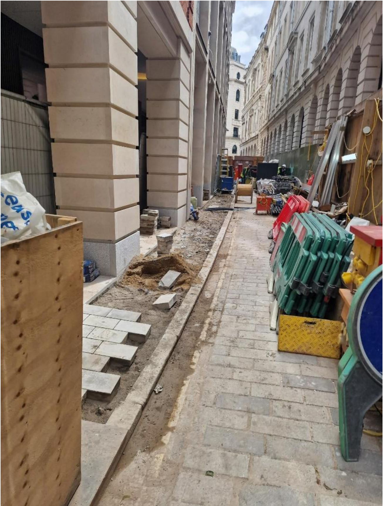
Ironmonger Lane | Hoarding to be removed to initiate improvements
